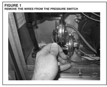
6. Disconnect the pressure switch hose which runs to the induced draft blower. (See Fig. 2).
