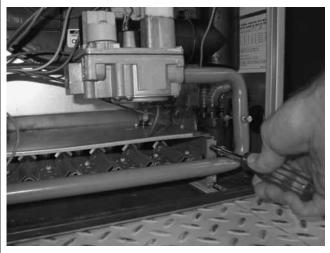
6. Remove the existing orifices from the manifold using a 7/16" socket or wrench. See Figure 7.
